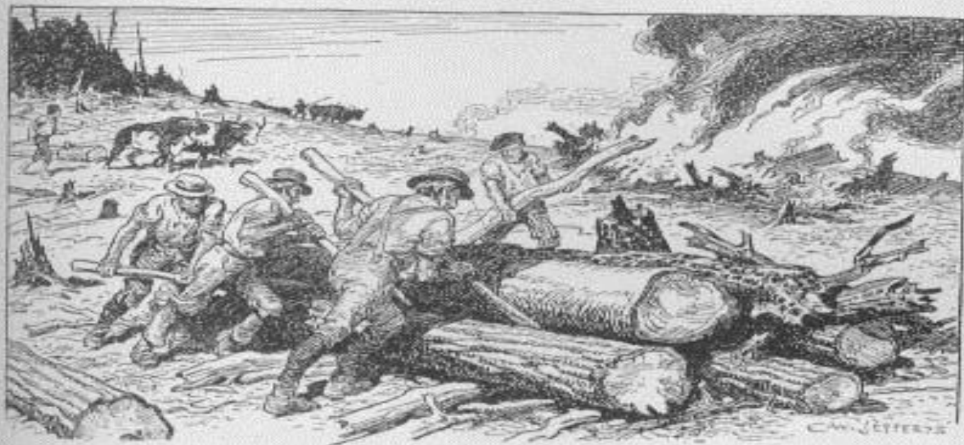
PILING LOGS AND BURNING
